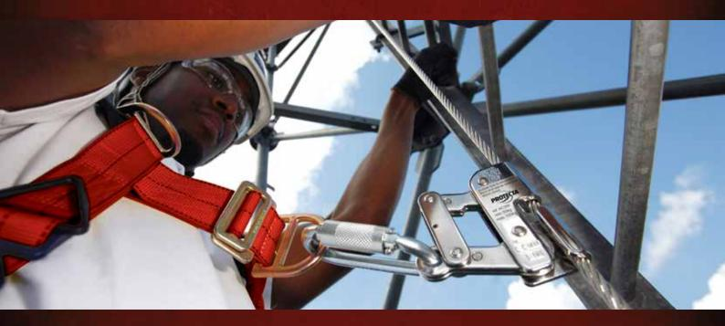
The Protecta® Cabloc™ vertical climbing system can be permanently installed to a ladder or other vertical structure that requires frequent access. It provides a safe, functional and practical means of access and egress.
