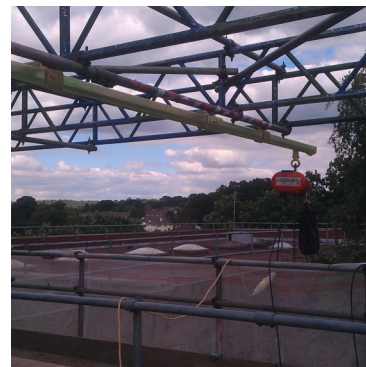
Scaffolding Runway Systems
