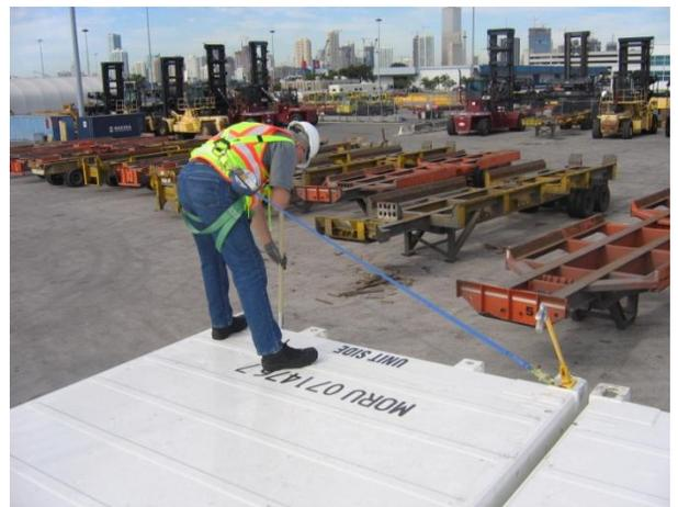
Worker working correctly one container width away and unlocking twist locks below with telescopic pole.
