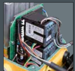
LOW VOLTAGE CONTROL
